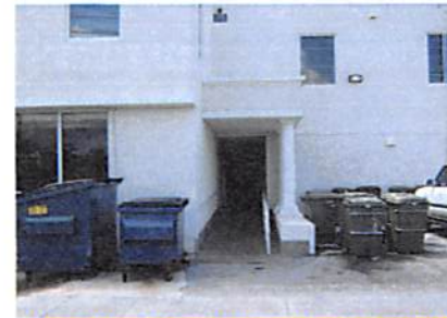
Figure 1-5: Existing Mid-Block Pedestrian Alley Proposed for Closure to Public
