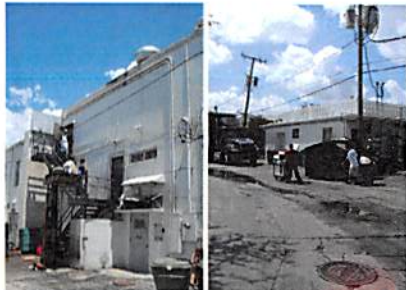
Figure 1-6: Existing Service Entrance
